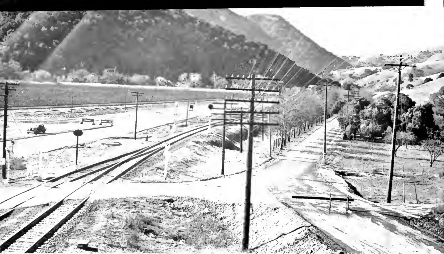
Old grade crossing west of Sunol, showing new highway on left beyond railroad crossing. Project eliminates three grade crossings
